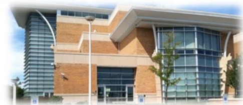
Aurora Branch Court 1200 East Indian Trail Road Aurora, Illinois 60505
