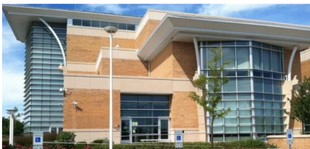
Aurora Branch Court 1200 East Indian Trail Road Aurora, Illinois 60505
